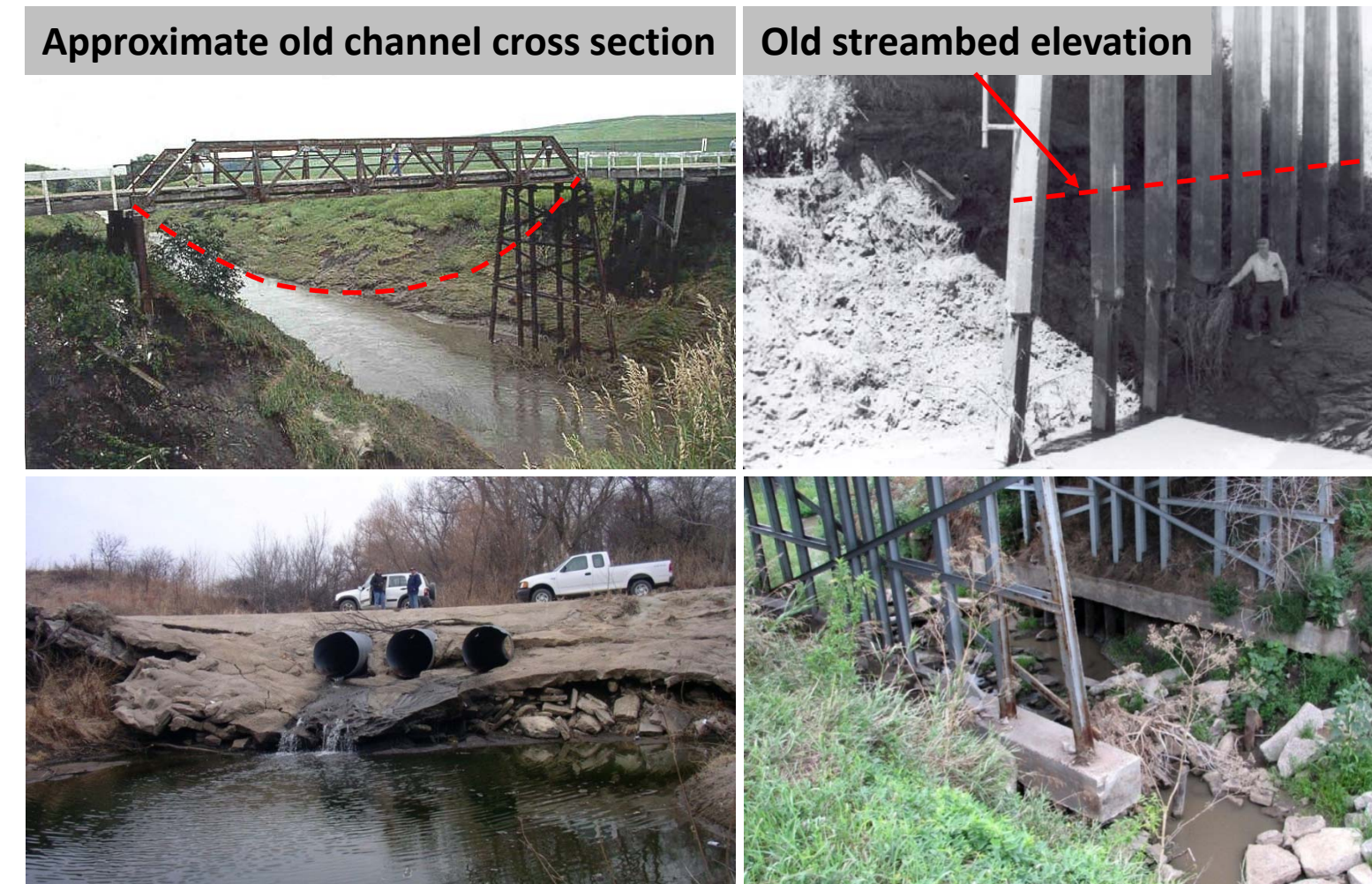
County road infrastructure damage due to streambed degradation
