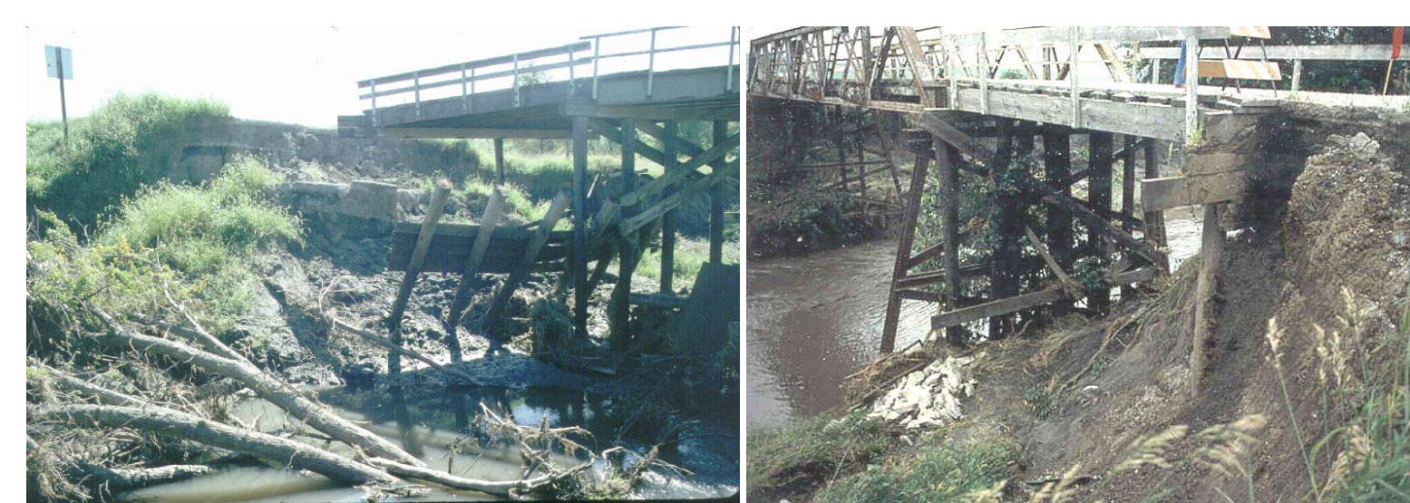
County road infrastructure damage due to streambed degradation
