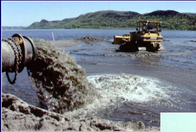
Constructing sand base with dredged material
