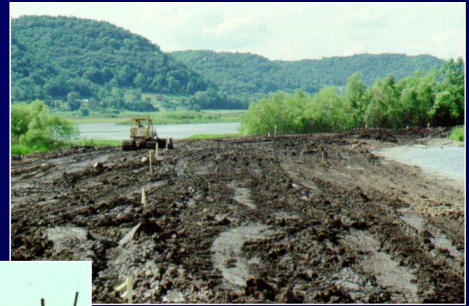
Shaping fine material (topsoil)
