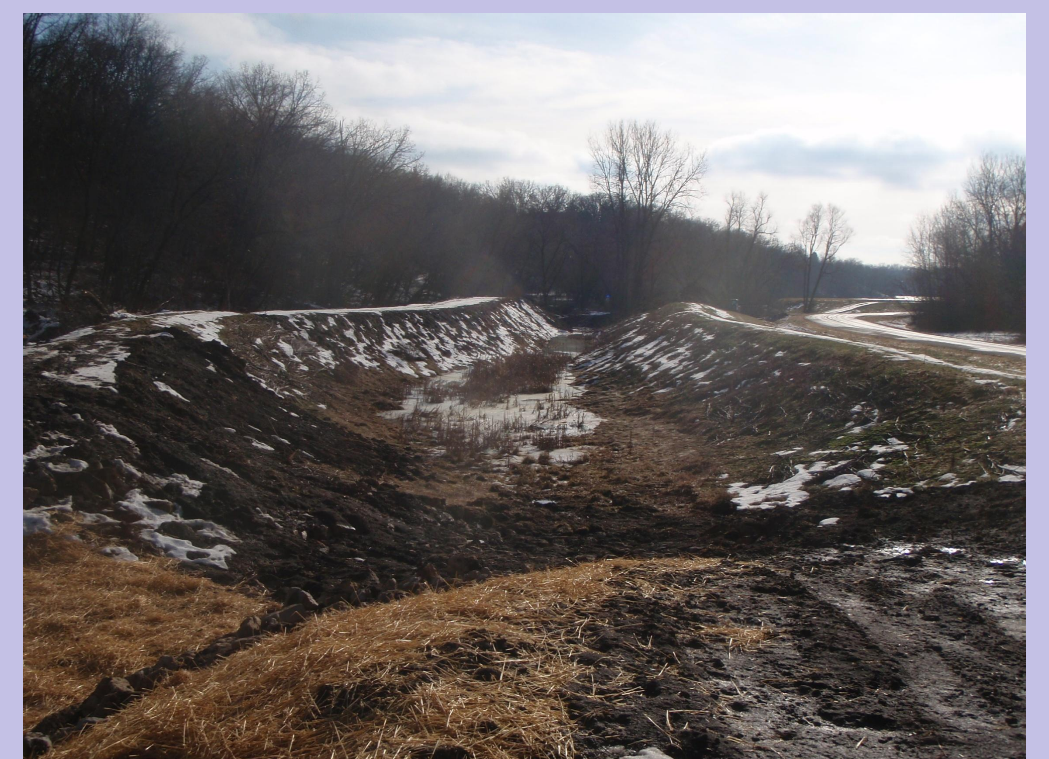
New wetland structure looking downstream.
