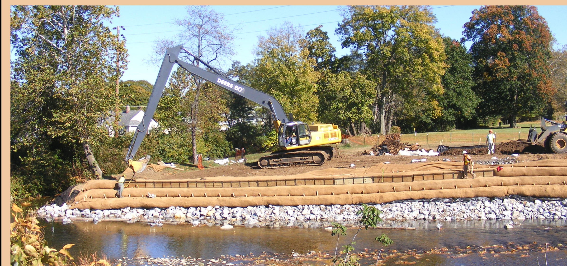
Rip rap at toe and three lifts of soil in place stabilized by coir fiber rolls.
