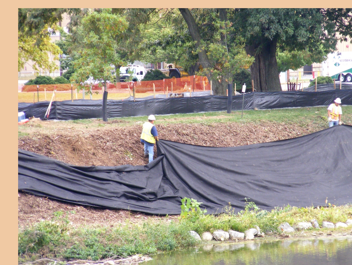
Vegetation cleared and filter fabric being placed to contain soil.
