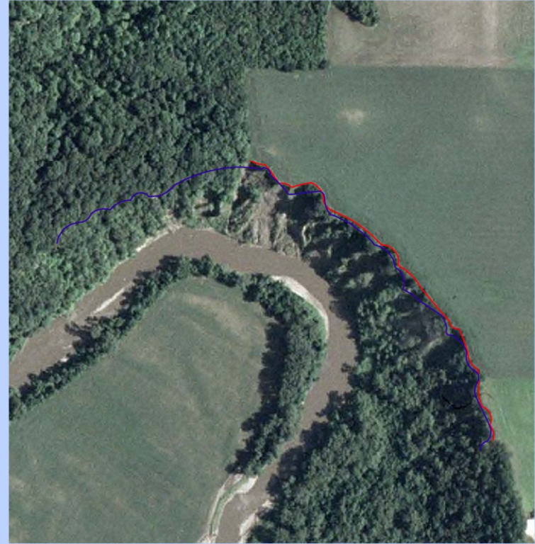
Bluff at intersection of Jansen Quarry on the LeSueur River
