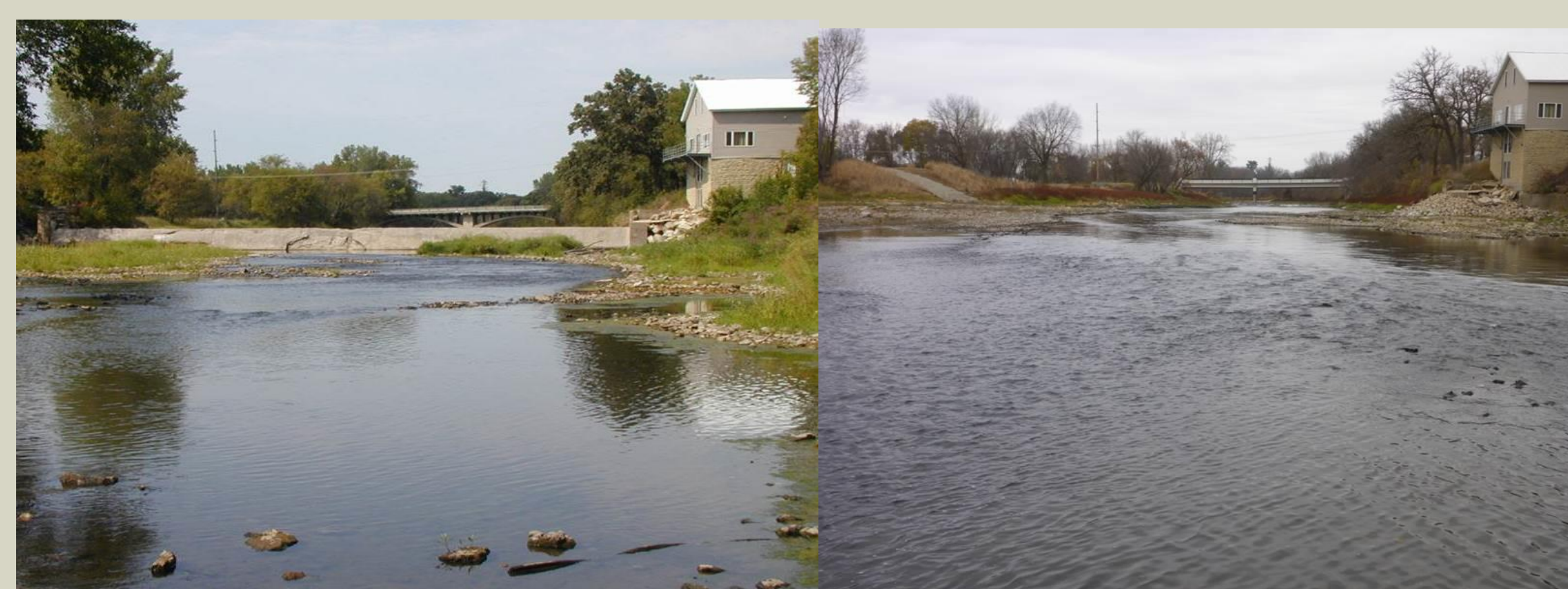
Figure 1. Shell Rock River at Rockford before and after removal of the dam.
