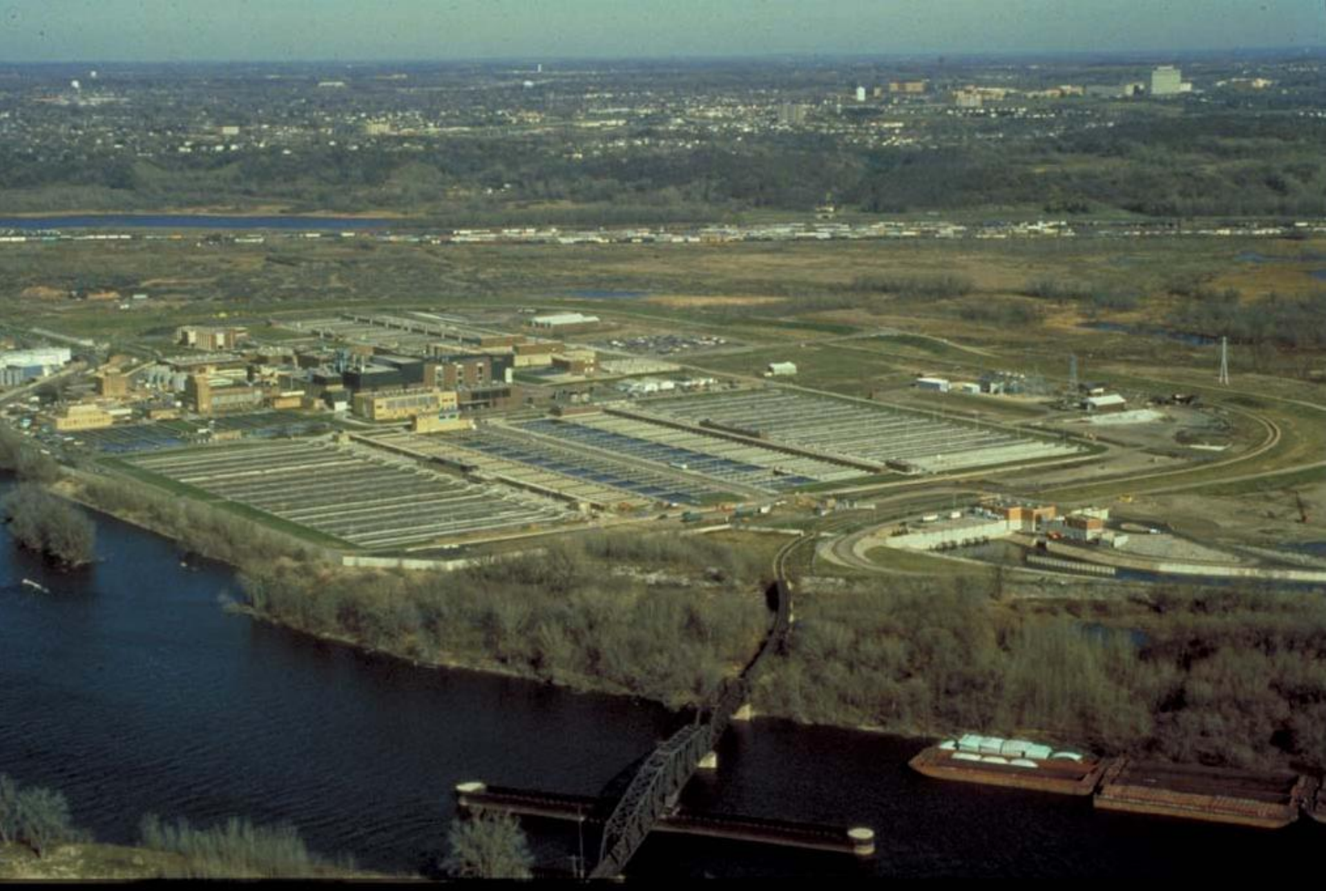
Metropolitan Wastewater Treatment Plant: ca. 1982
