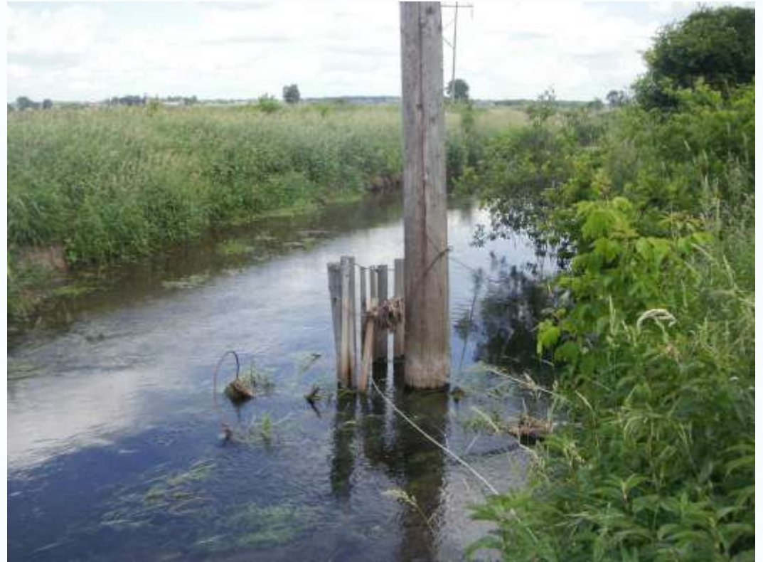
Photo. View downstream exposed pole structure (Summer 2011).
