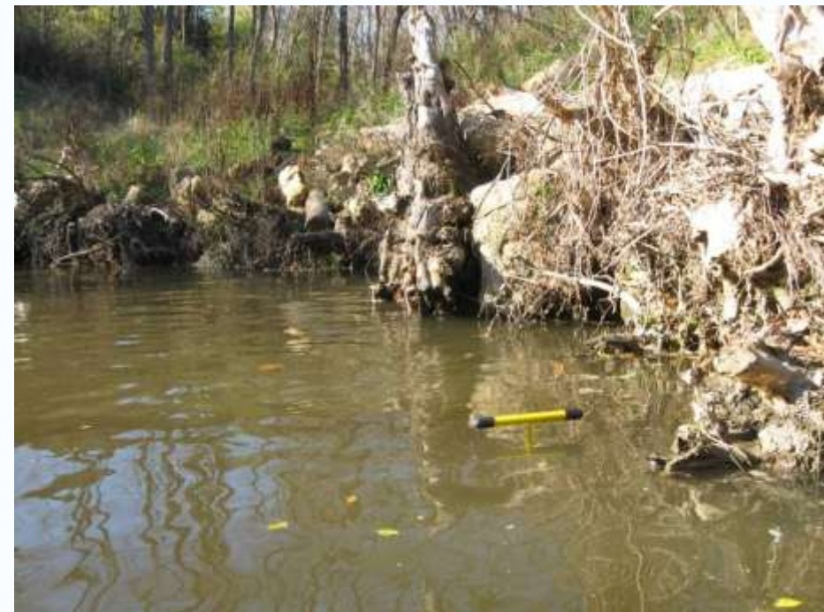
Photo. View upstream scour pool in front of rootwad revetments.
