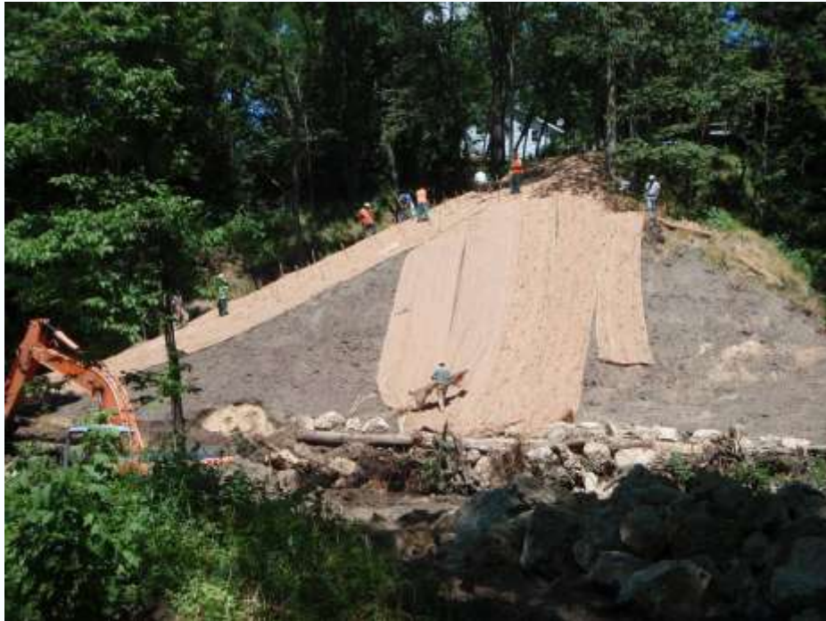
Photo. View at the graded slope during erosion control blanket installation.
