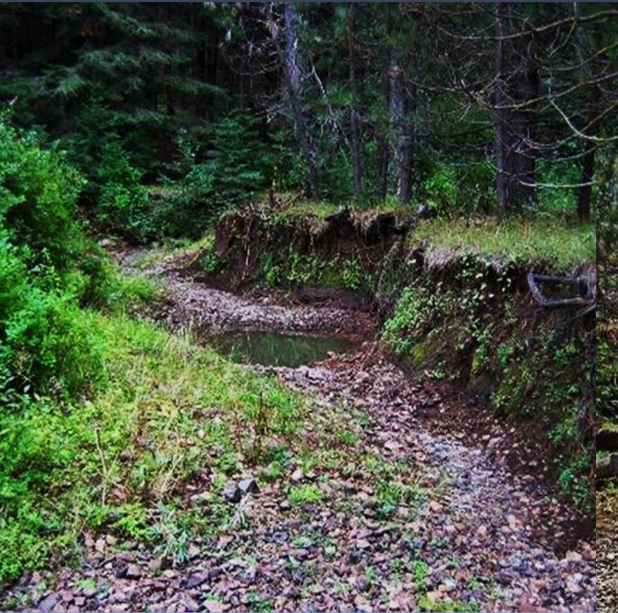
Channel raised 3ft to reconnect the river with its floodplain
