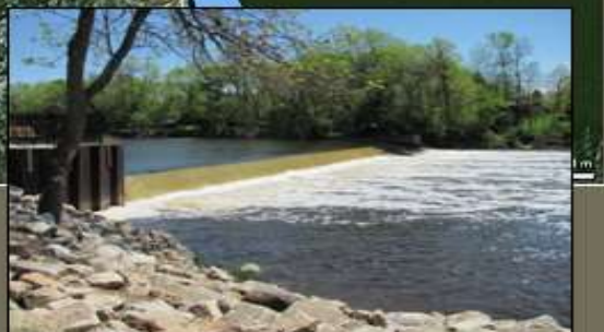
The Mequon-Thiensville Dam, no longer an impediment to native fish passage
