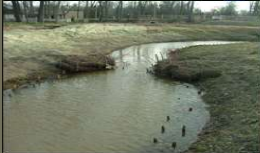
Pools above each rock weir, allowing fish to rest and continue swimming upstream
