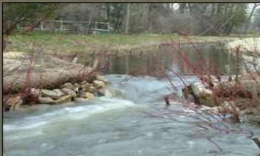
One of eight rock weirs that allow fish to move through the fishway elevation change
