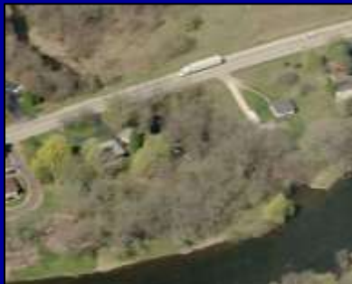
Mole Creek/CTH O Culvert Replacement (2012)
